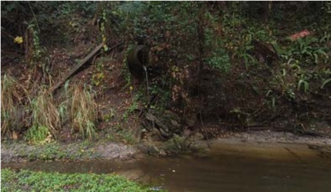
Photo ID# 062421000015MW – 18” RCP from Dogwood Ct on north bank of River (Echo, 2021)
