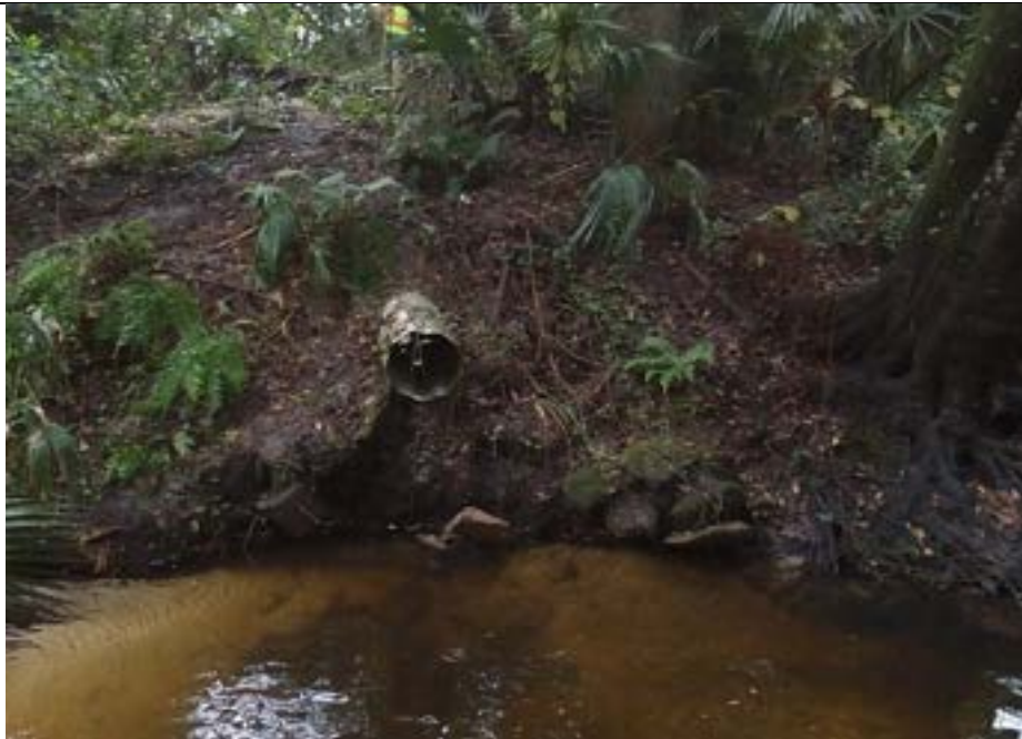
Photo ID# 062421000013MW – 24” RCP from Forest Ct east of Northwestern drive on N bank (Echo, 2021)
