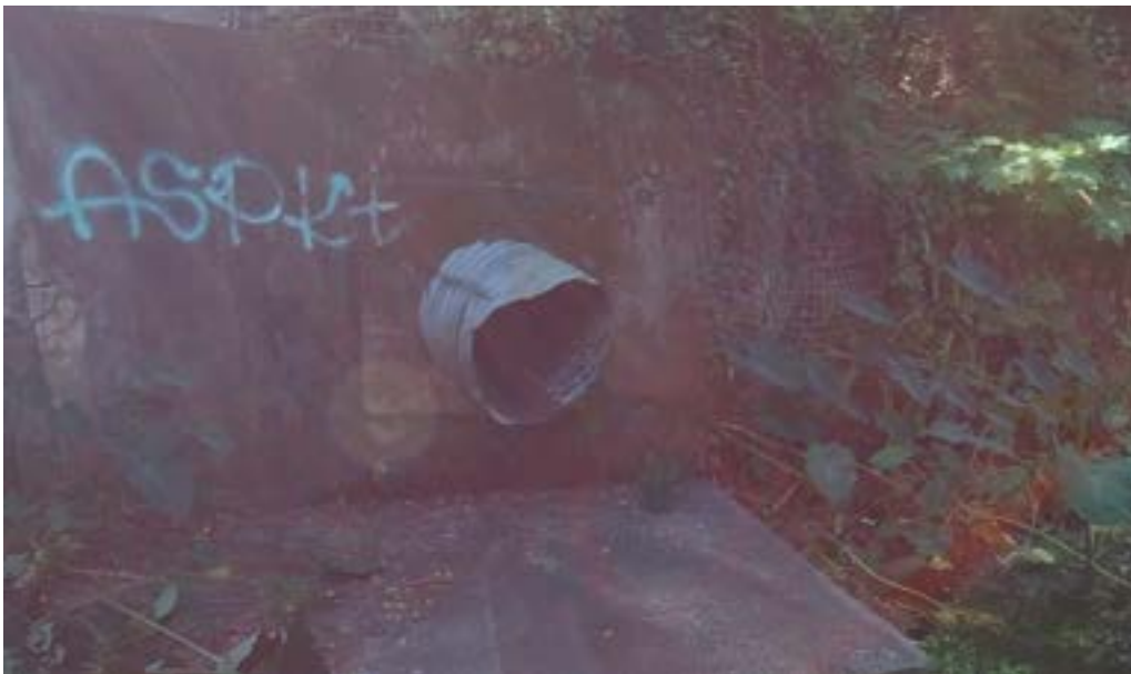
Photo ID# 062421000022MW – 24” CMP at Weathersfield Avenue bridge on north bank of River (Echo, 2021)
