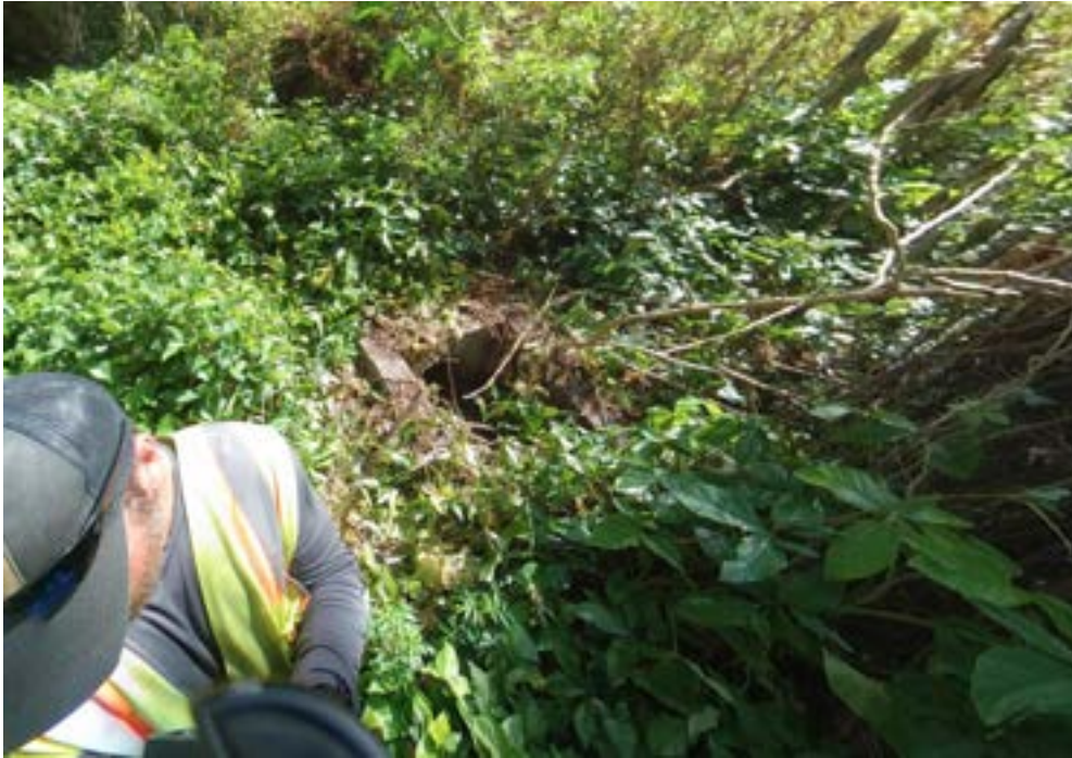
Photo ID# 062421000011MW – 24” RCP MES from Little River Loop upstream of SR 434 (Echo, 2021)
