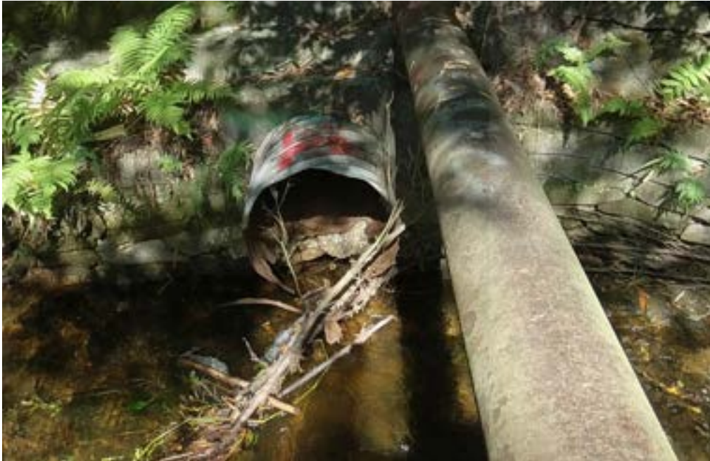
Photo ID# 062421000022MW – 24” CMP at Weathersfield Avenue bridge on north bank of River (Echo, 2021)
