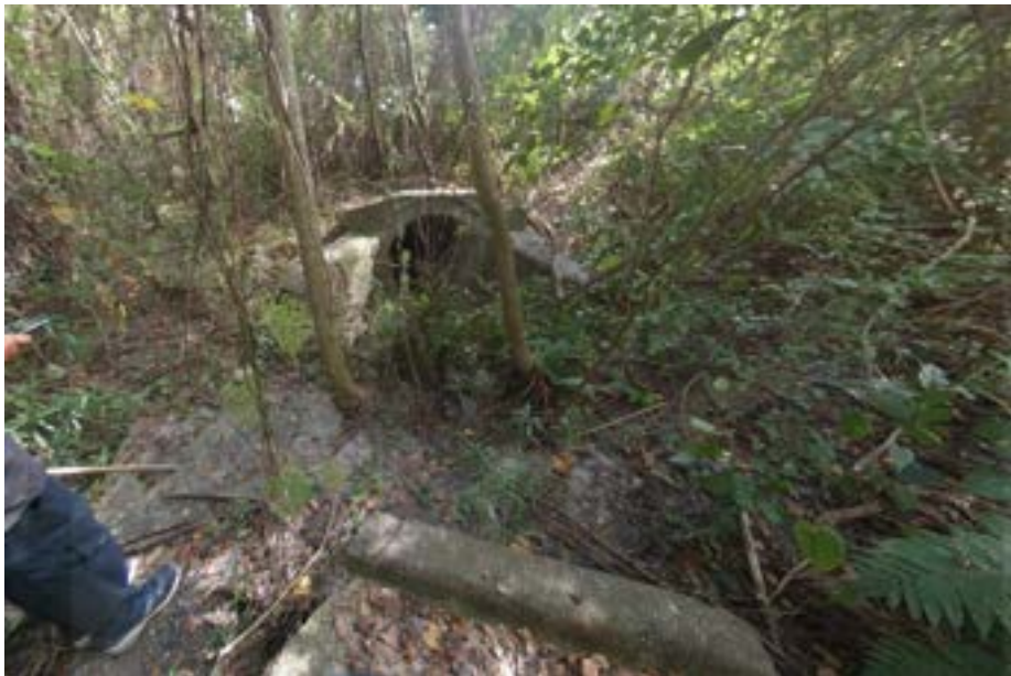
Photo ID# 062421000001MW- 36” RCP Wing Wall on S bank of Trout Lake (Echo, 2021)
