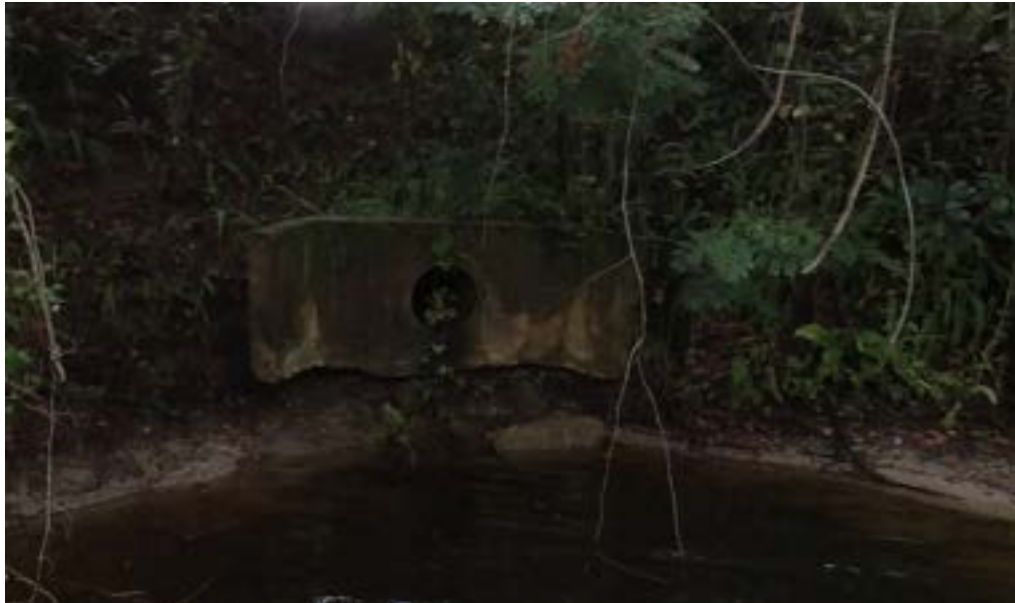
Photo ID# 062421000017MW – 24” RCP from Moss Drive on north bank of River (Echo, 2021)
