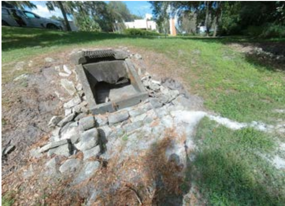
Photo ID# 062421000008MW – 18” RCP Control Structure on NNW bank of Trout Lake (Echo, 2021)
