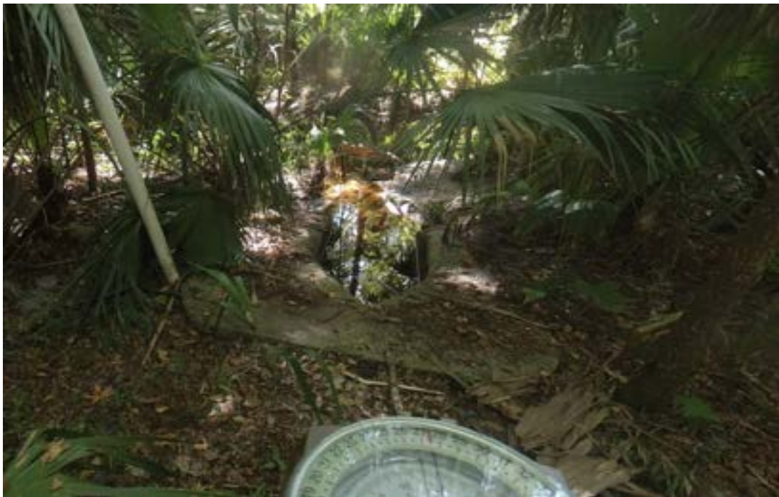
Photo ID# 062421000110MW – 19” x 30” ERCP MES from Biltmore Point (Echo, 2021)
