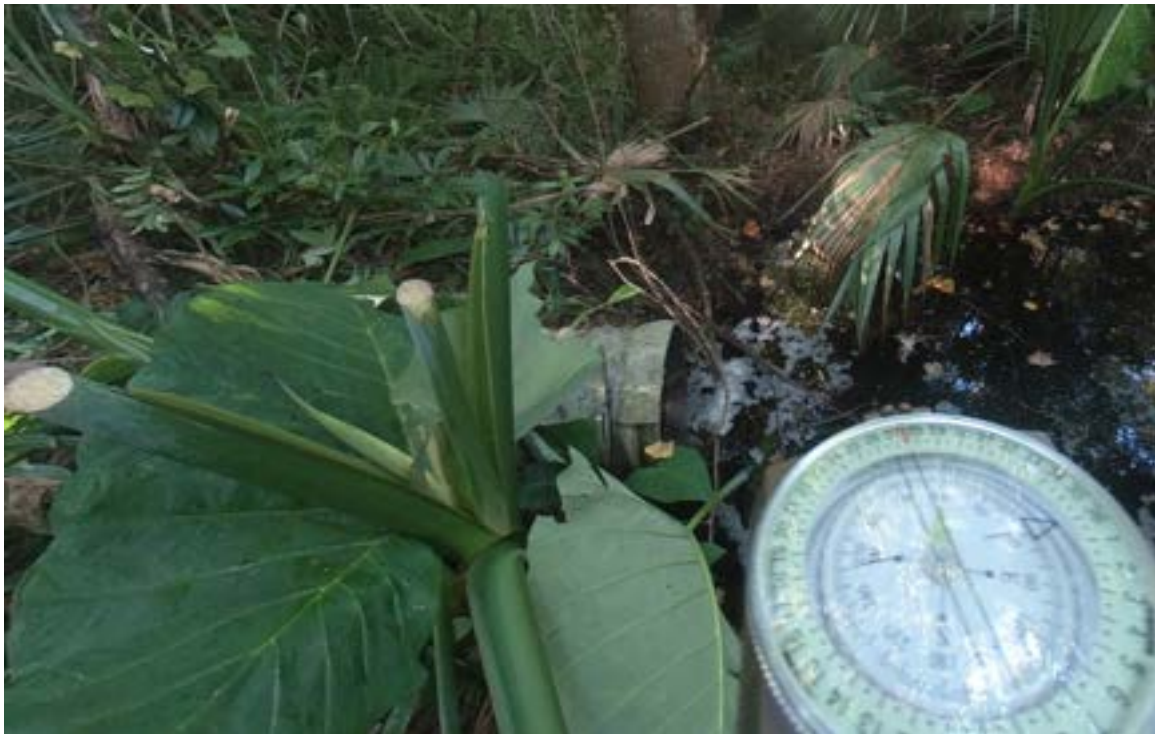
Photo ID# 062421000108MW – 15” CMP near Riverpark Circle (Echo, 2021)
