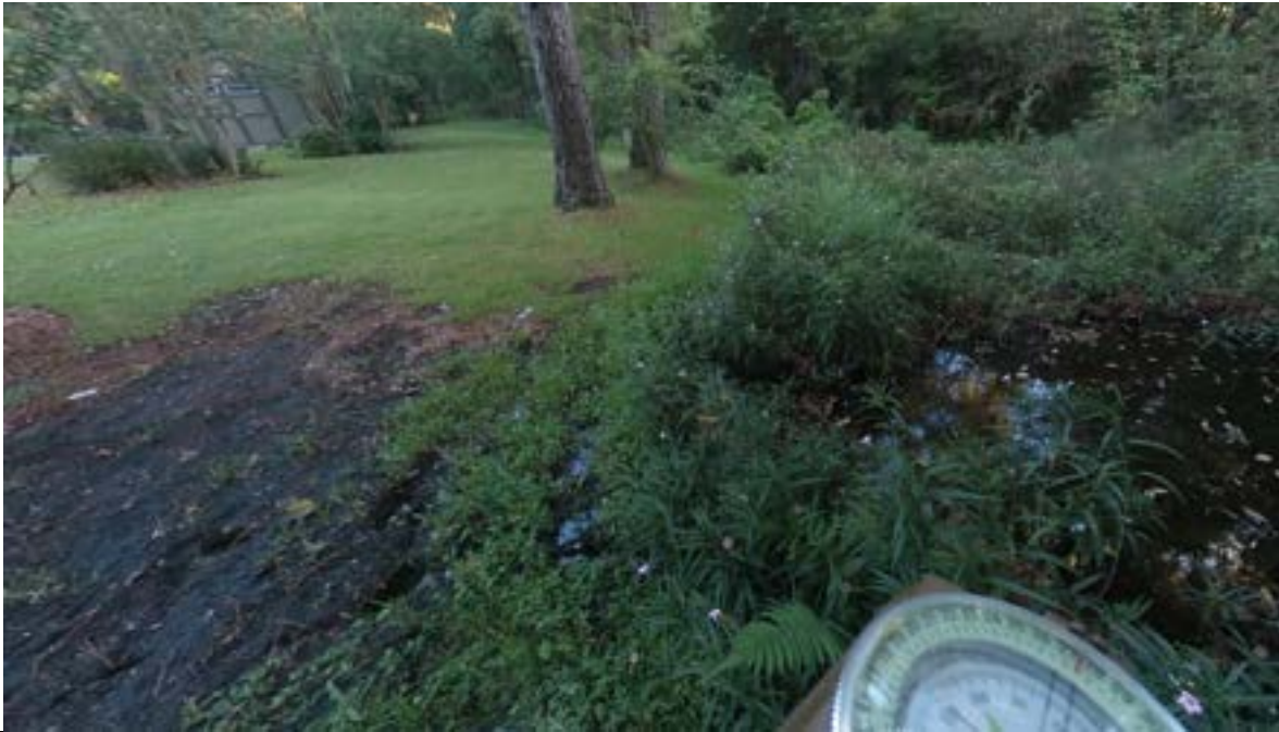
Photo ID# 062421000107MW – 24” RCP from Riverpark Circle (Echo, 2021)
