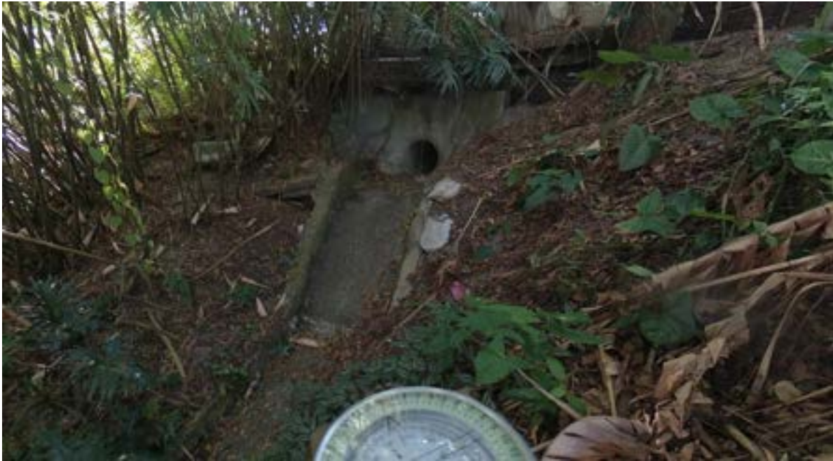
Photo ID# 062421000005MW – 18” RCP from Pine Ct on south bank of River (Echo, 2021)
