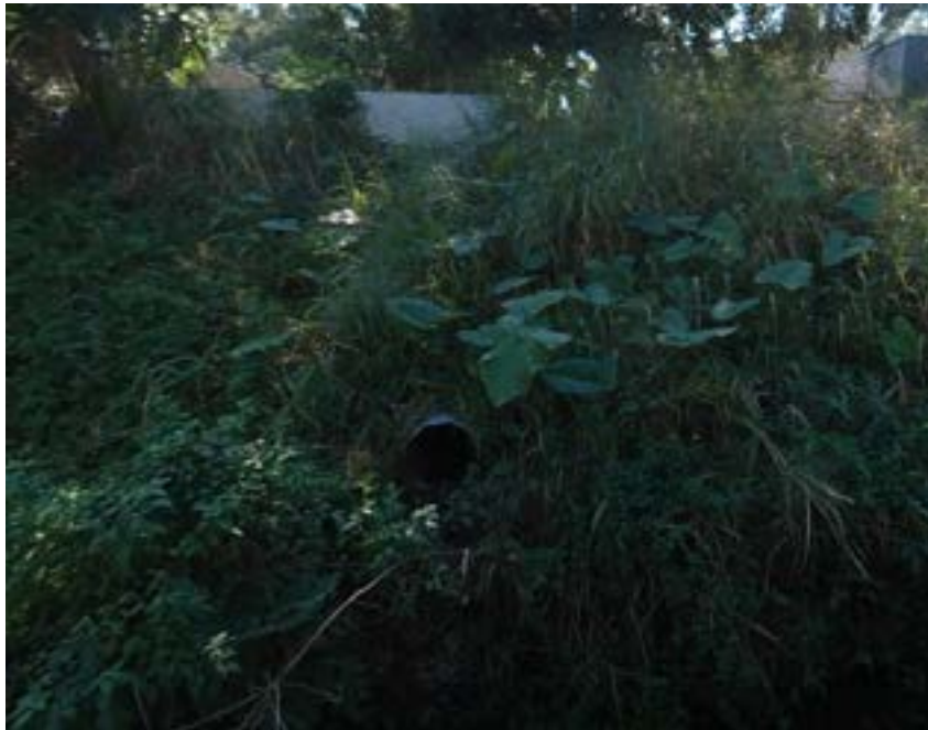
Photo ID# 062421000020MW – 18” CMP from Variety Tree Cir on SW bank of River (Echo, 2021)
