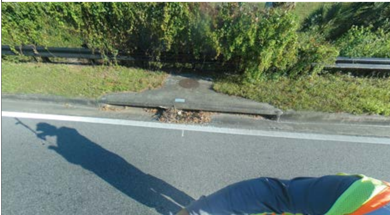
Photo ID# 062421000024MW – Manhole and curb inlet connecting 15” RCP (S), 18” RCP (W), and 15” RCP (E) on Orange Avenue (Echo, 2021)
