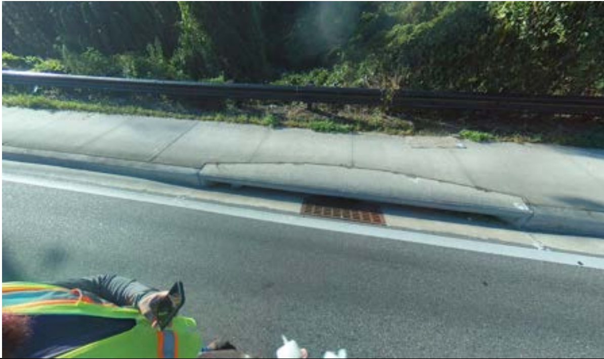
Photo ID# 062421000116MW – 15” RCP curb inlet on Orange Avenue (Echo, 2021)
