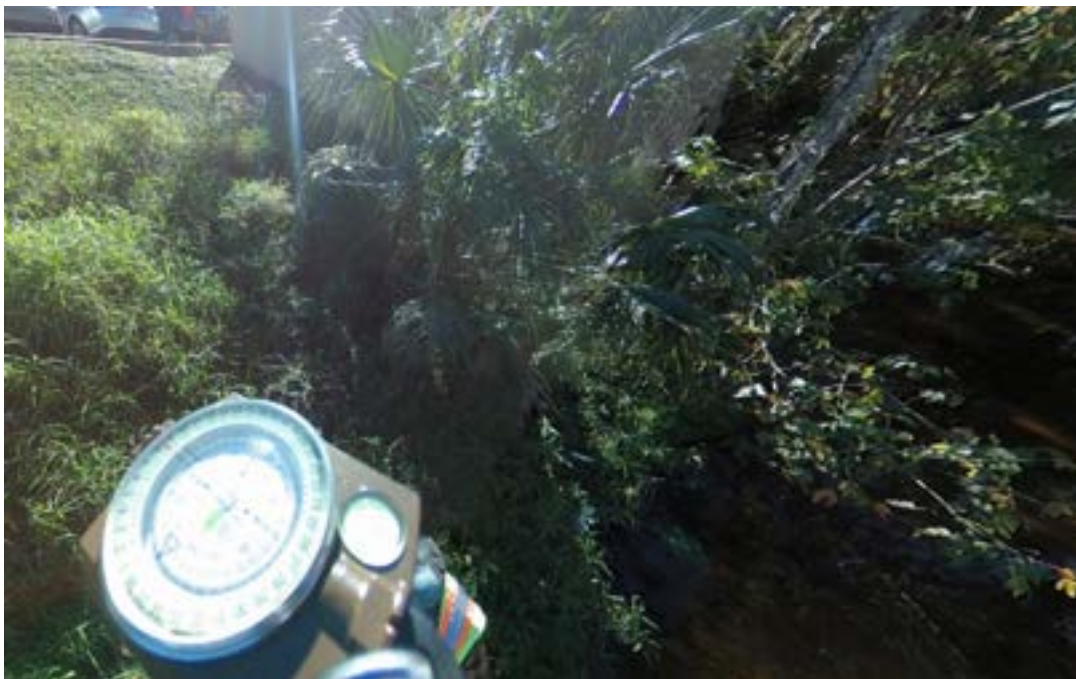
Photo ID# 062421000009MW – 15” RCP MES on W bank of Trout Lake (Echo, 2021)
