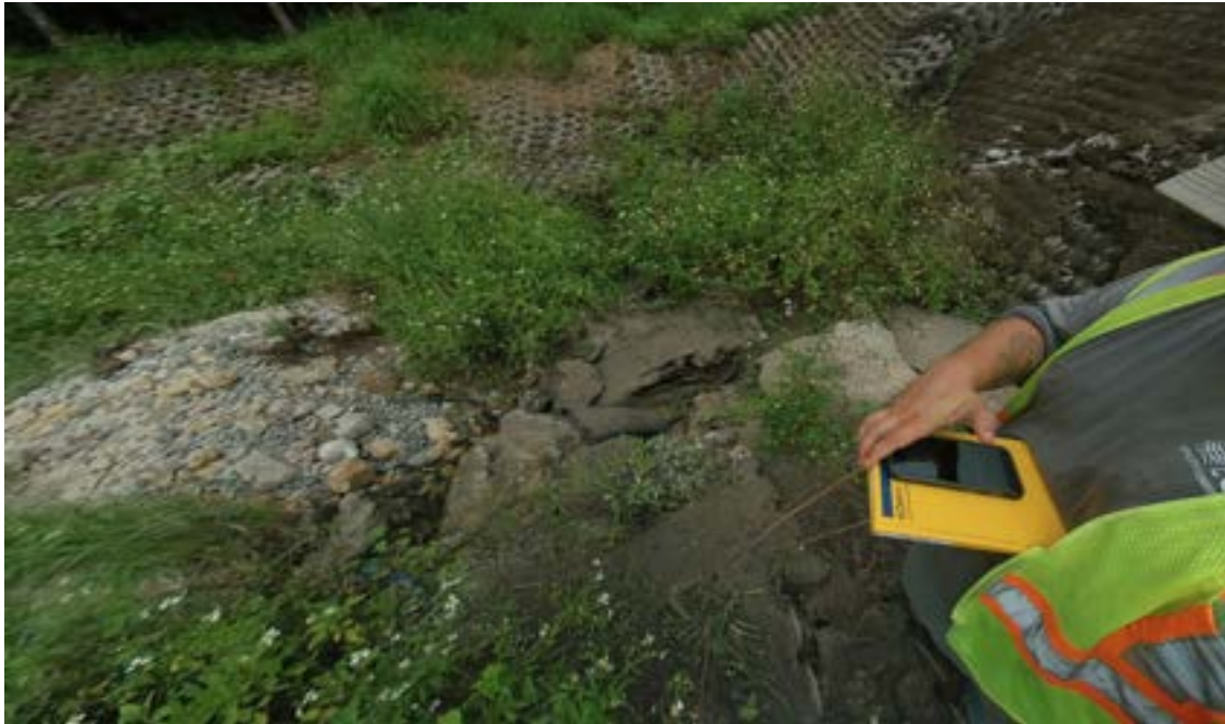
Photo ID# 062421000124MW – 18” RCP from SR 434 (Echo, 2021)
