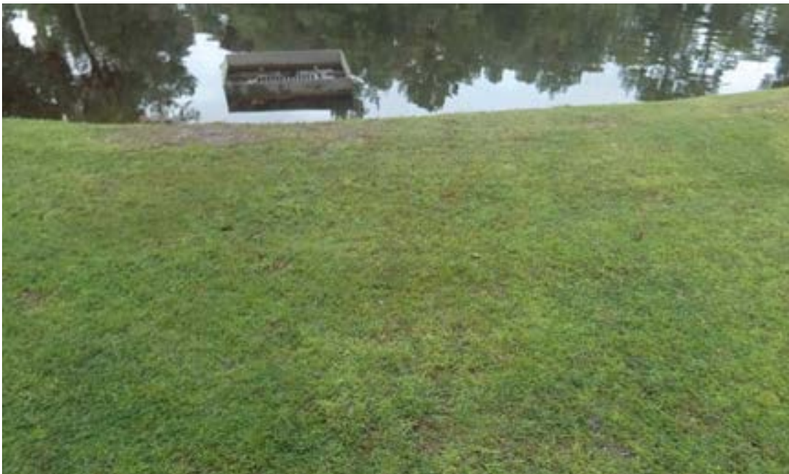
Photo ID# 062421000105MW – 15” Pipe from pond north of Spring Landing Blvd (Echo, 2021)
