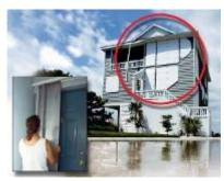
Installing storm shutters on windows, sliding glass doors, skylights, and French doors is one of the best ways to protect your home. You can buy manufactured shutters made of wood, steel, or aluminum. You can also make storm
